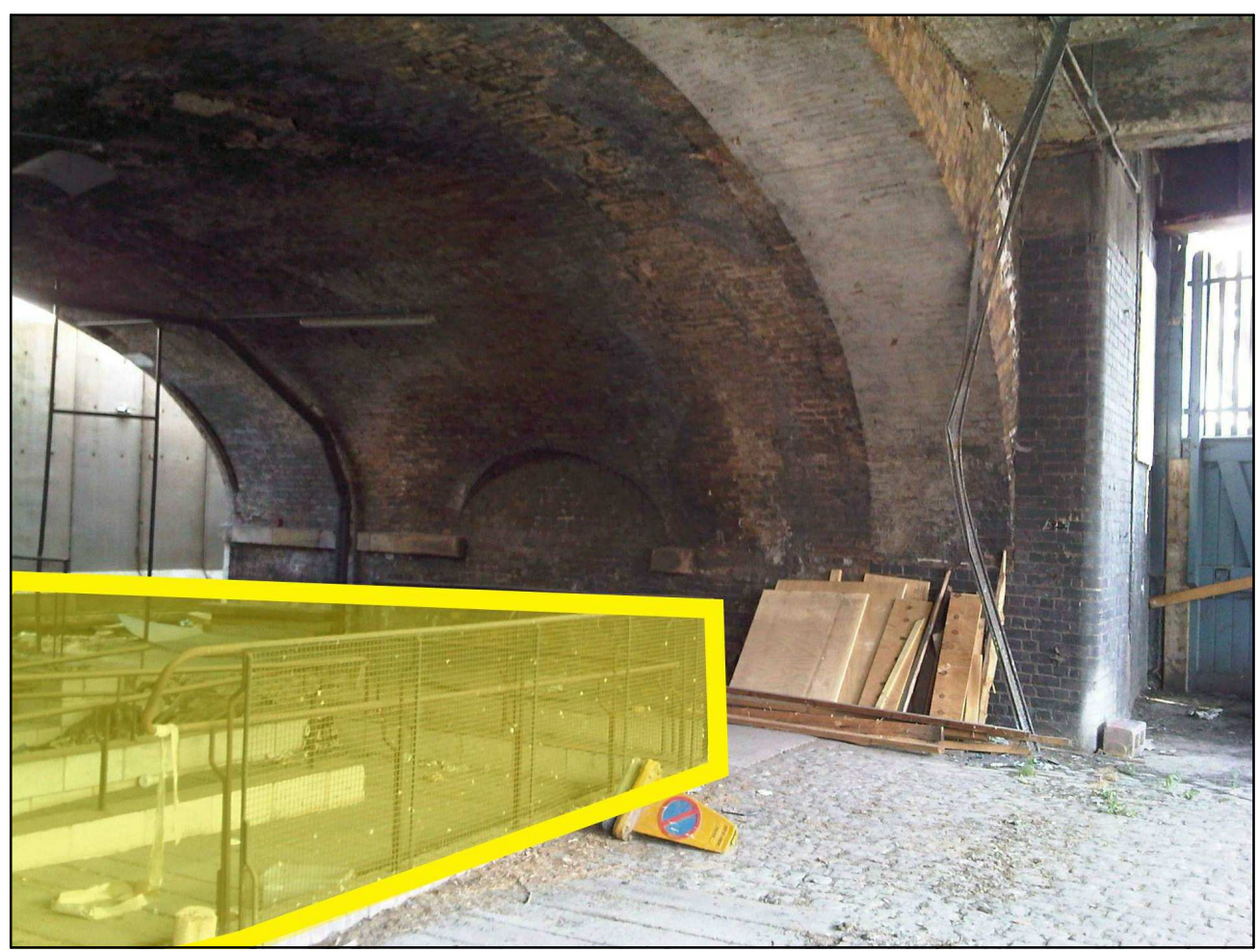
FINAL ARCH ADJACENT TO BRICK LANE BOUNDARY WALL - Ramps highlighted to be removed to provide level access to retail unit
